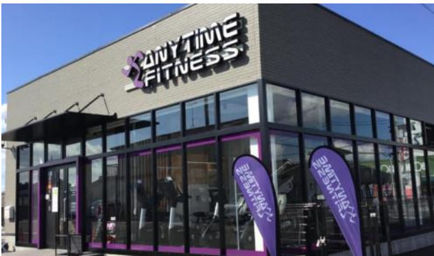
Figure: Exterior view
